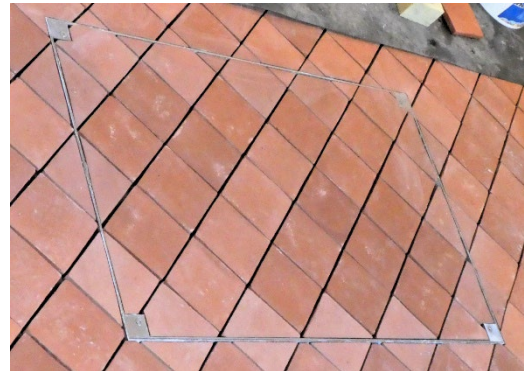
Tiling over a manifold cover:
